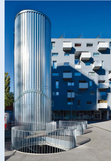
▶ 200 m 3 energy storage tank (Source: Fotohof)
