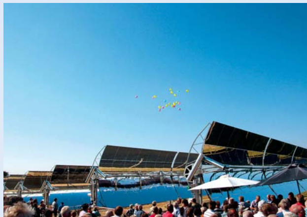
▲ Opening of the Taars solar thermal system (Source: Aalborg CSP)
