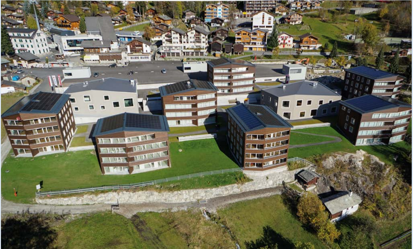
▲ Aerial view on the “Reka Feriendorf” in Naters, Switzerland (Source: Lauber IWISA AG)
